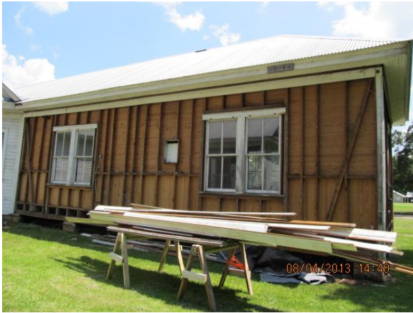
Renovation - south wing
